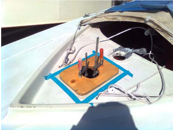
.. mast partners clamped in place...
