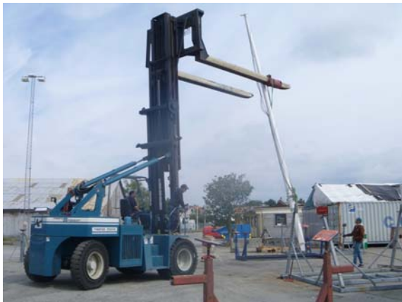
15:11, another lift picks up the mast...
